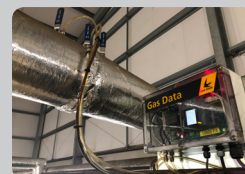
Gas Flow Monitoring
